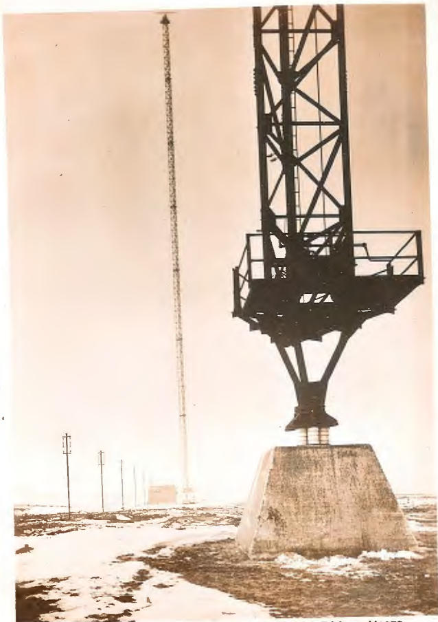
NORTH REGIONAL STATION. BASE OF ONE OF THE 500 FT. MASTS. B.B.C. COPYRIGHT
